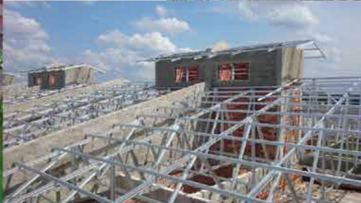
60unit shoptot Triang, Pahang TH Truss
